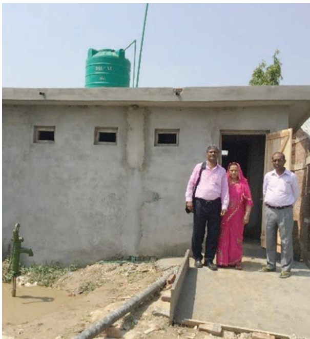
Construction of additional toilet for girls
